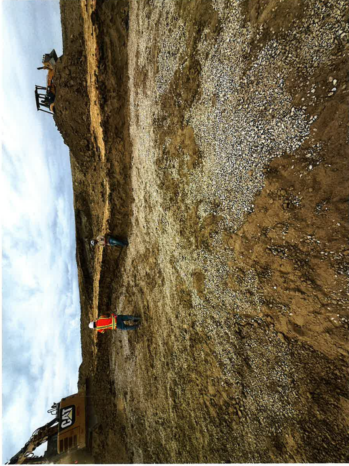
Began construction on Oct 16. Peeling off existing dirt and top layer of existing fabric to expose existing drain rock.
