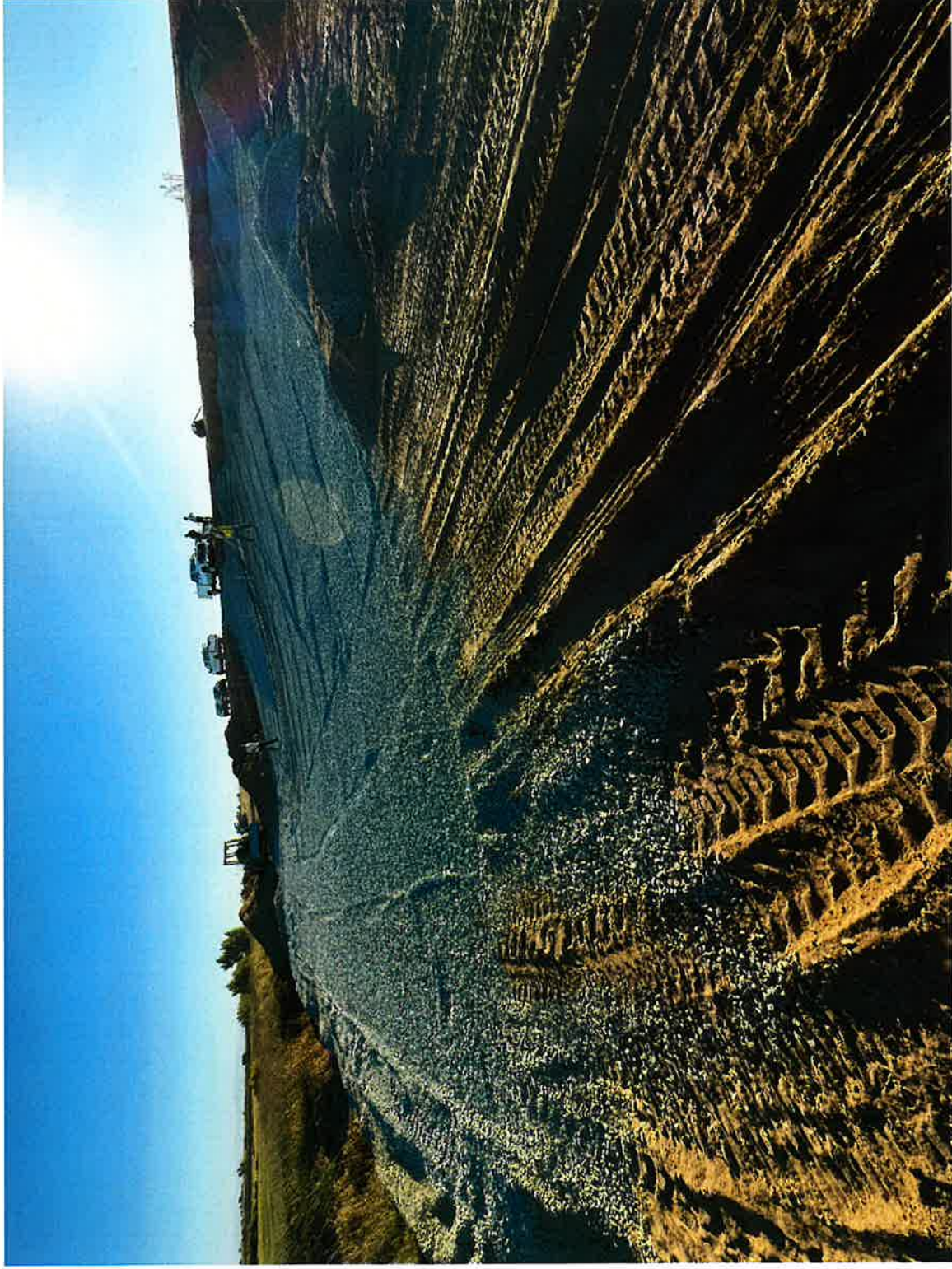
All new drain rock has been placed.
