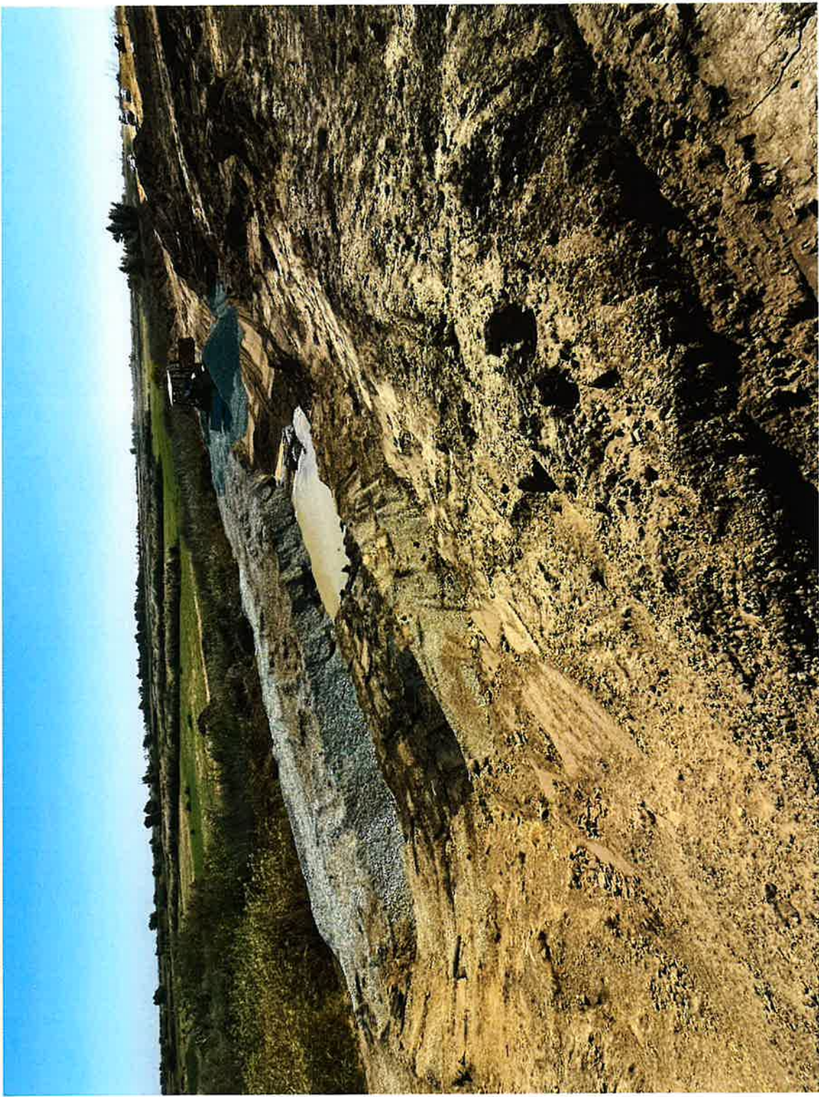
All existing drain rock and bottom layer of existing fabric on second pass have been removed. Placing new filter sand and drain rock.
