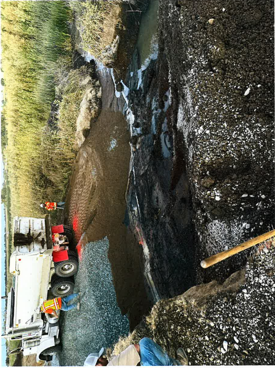
Placing new filter sand and drain rock.
