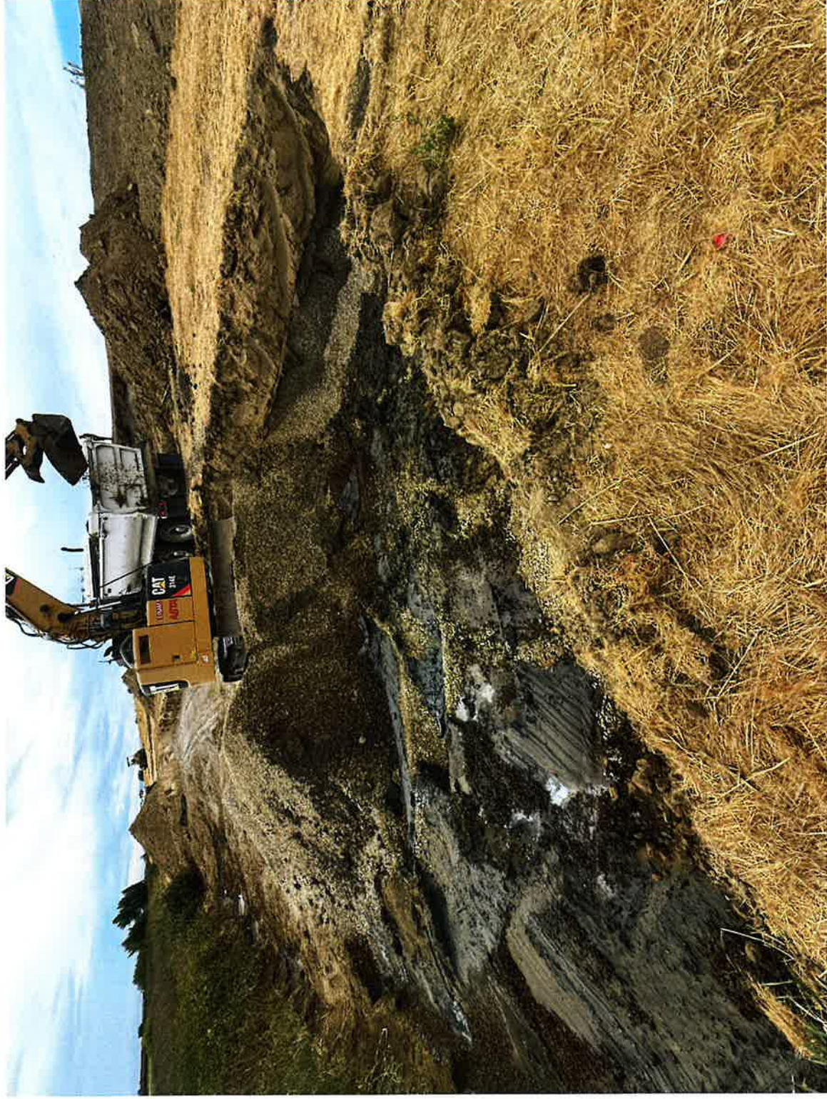
Removing existing drain rock and bottom layer of existing fabric.
