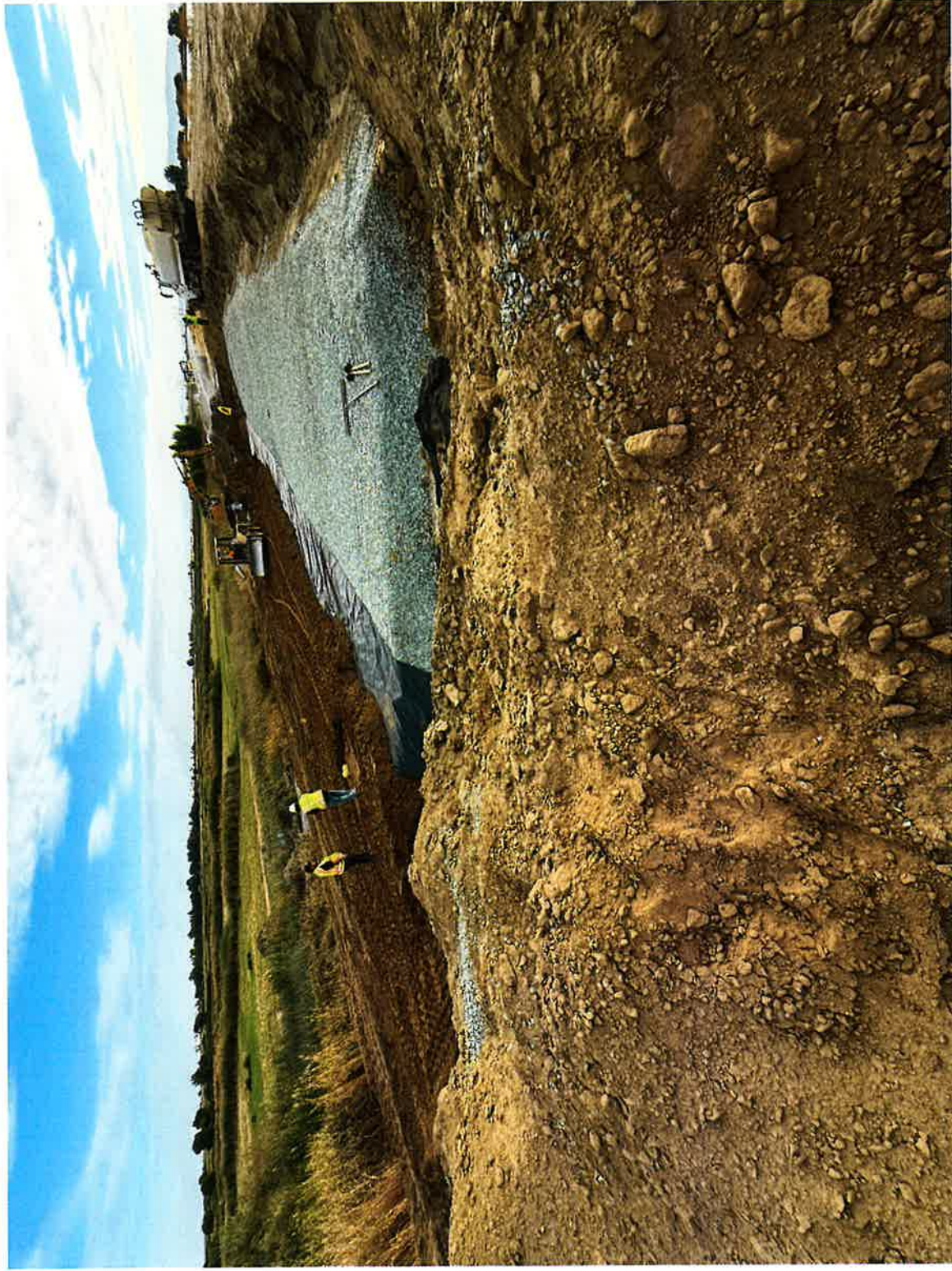
Placing new fabric and fill material.
