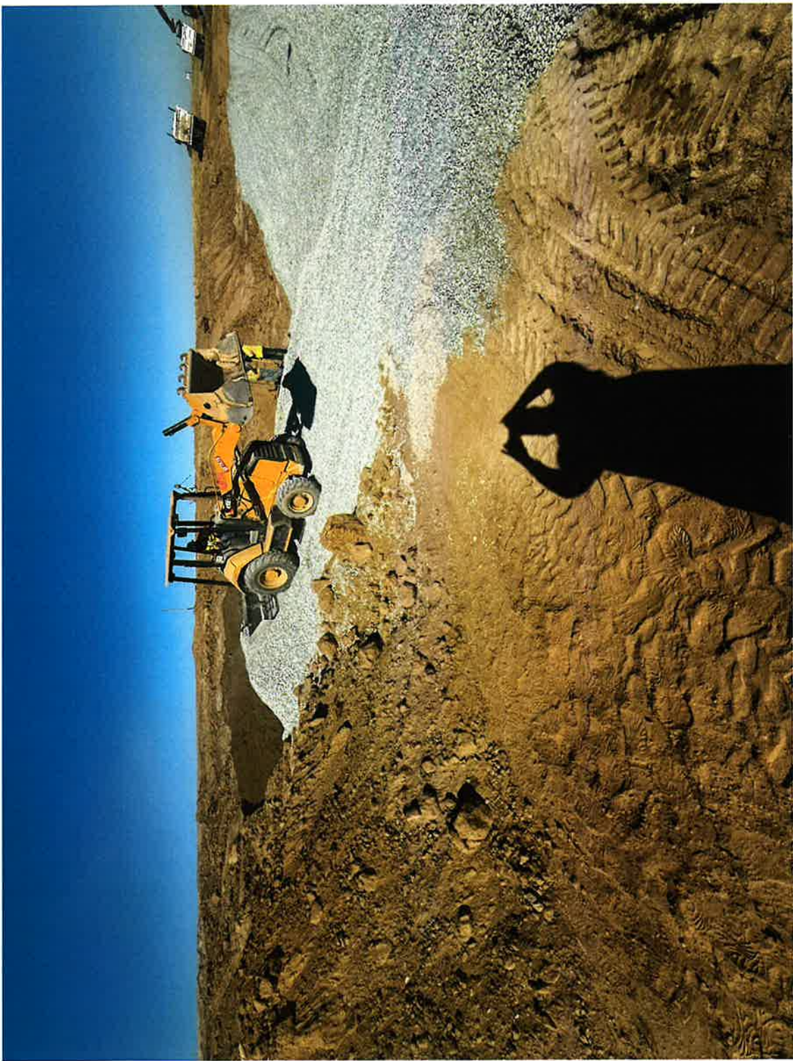
Placing new filter sand and drain rock at levee slope.
